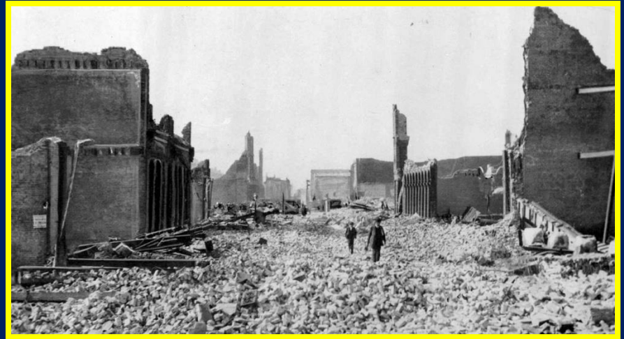
1906 San Francisco Earthquake 7.9
