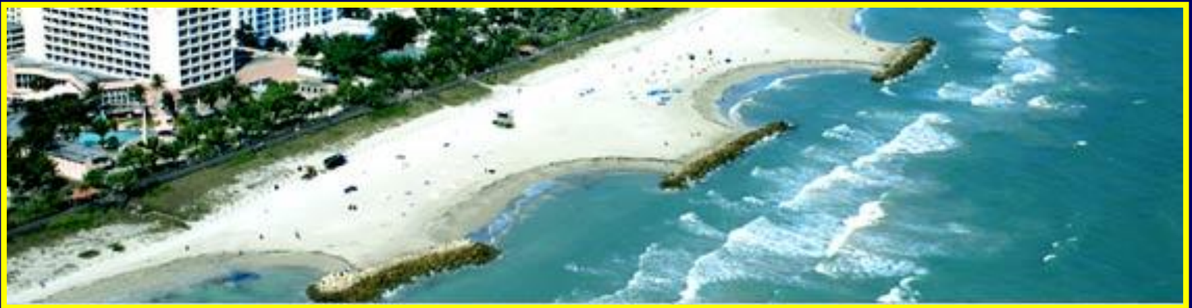
Series of Breakwaters in Miami, Florida.
