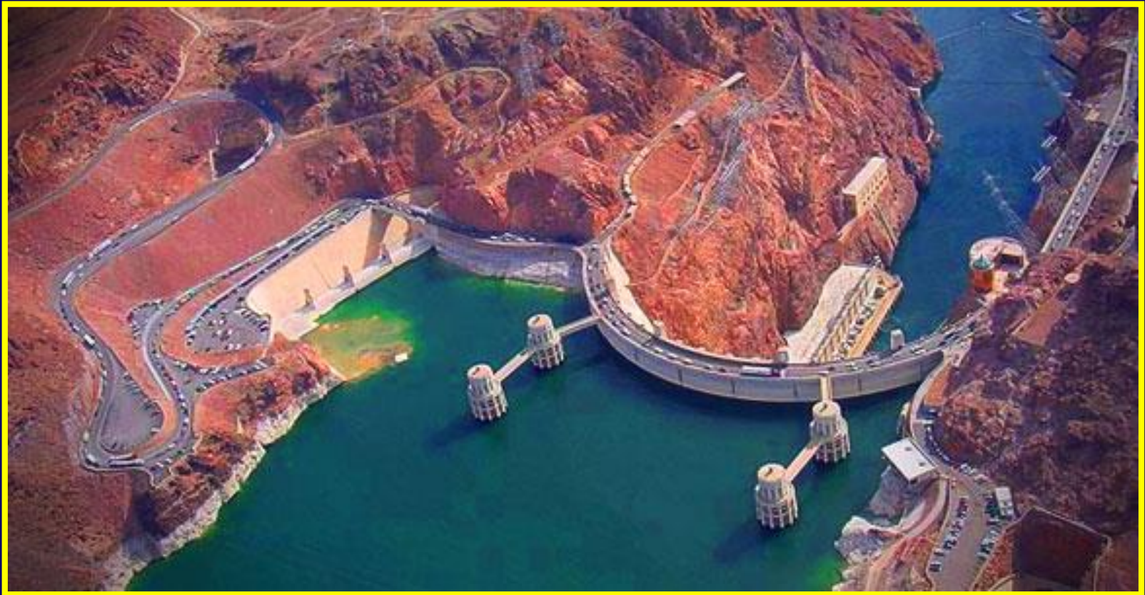
Hoover Dam on the border between Arizona and Nevada
