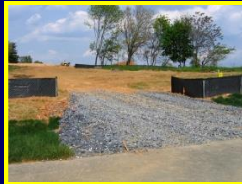
Gravel at Entrances
